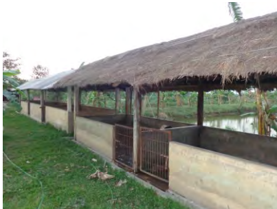
Pig sty over the pond embankment
